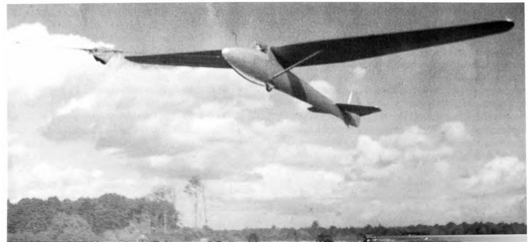
BGA 663 being given a winch launch at Lasham in 1951. The pilot is Ralph Hooper. The only hook provided was in the nose, the advantages of a rear hook mounting not having
